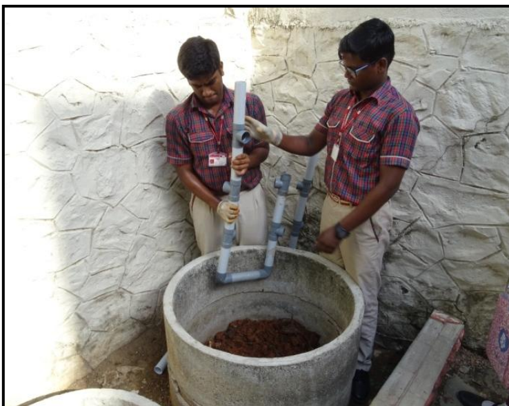
Fitting Pipes in the Compost Pit
